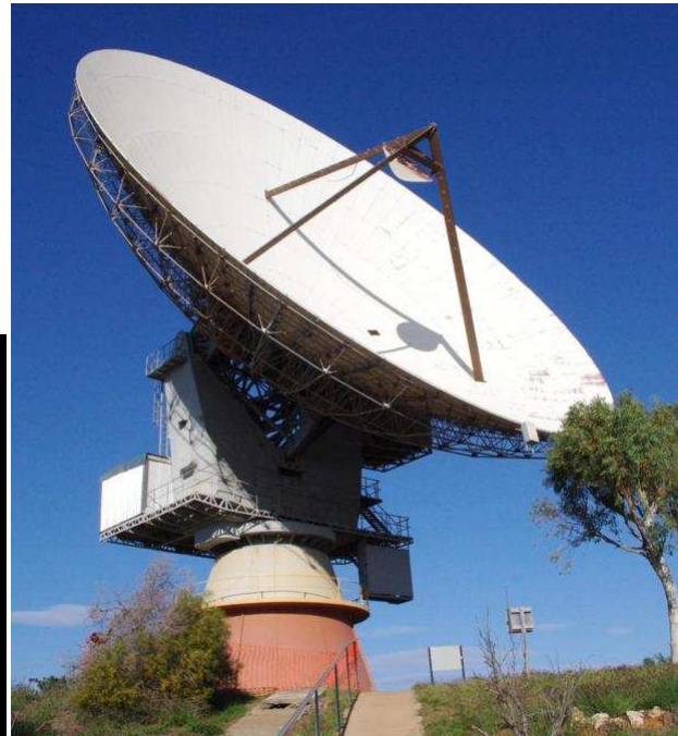
Carnarvon's OTC dish (Earth tracking station) was built in conjunction with NASA in 1966 as a satellite communications & tracking station. The station was involved in the Apollo space missions. The dish is 29.6 metres in diameter & weighs 300 tons & is no longer used. All the original NASA buildings have been removed.
